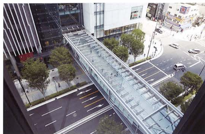
南館・北館 接続デッキ(2階) The second-floor deck connecting the South Building and North Building
