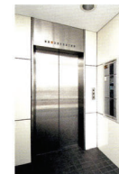
● 1F EV HALL
