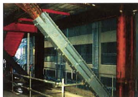
制震ダンパー Anti-earthquake damper
