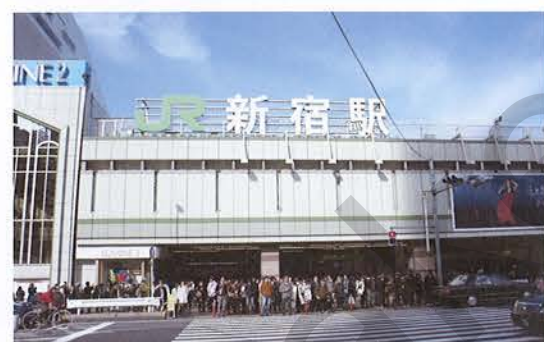
JR新宿駅南口 JR Shinjuku Station South Exit
