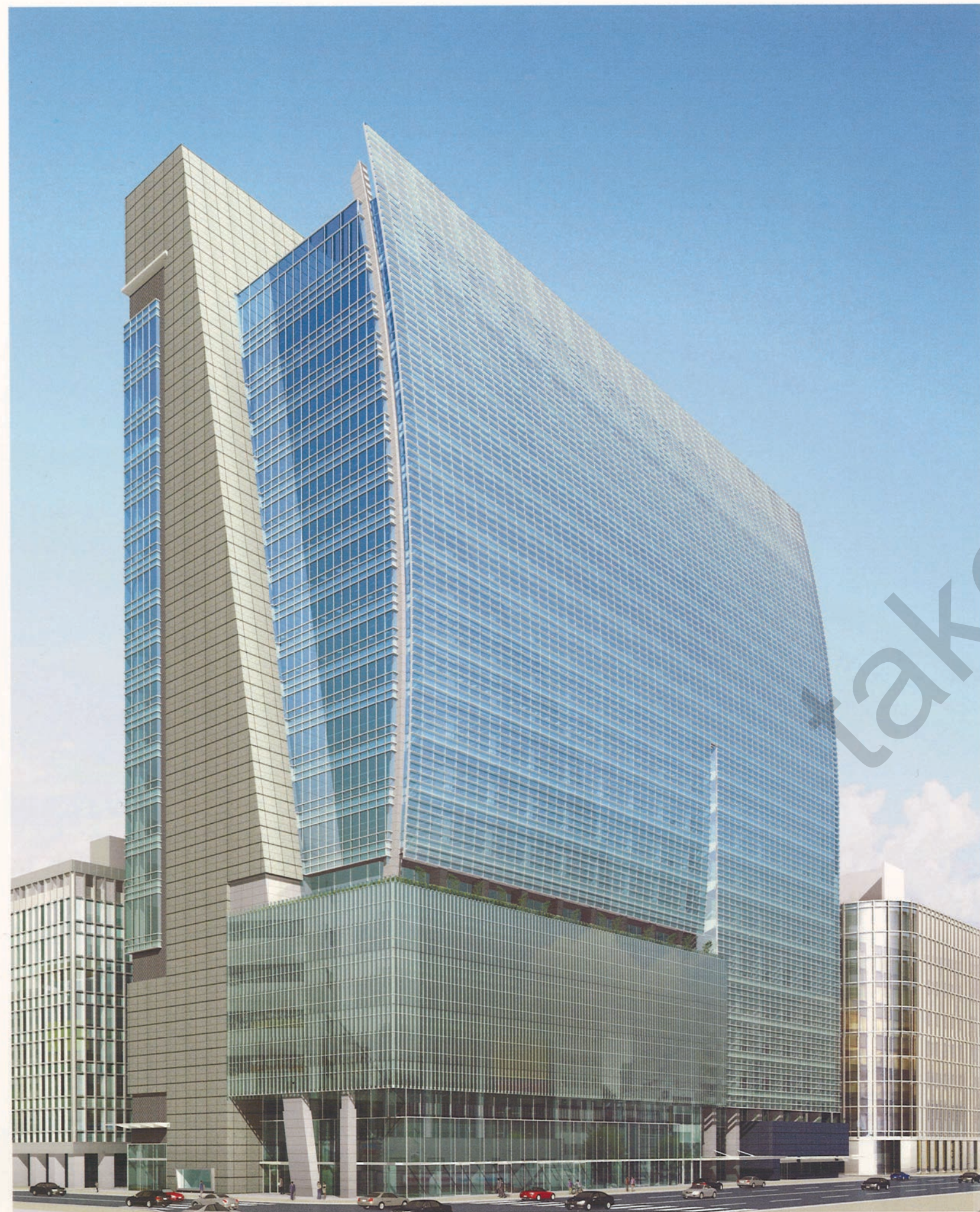
日本橋交差点から Image of the completed building, viewed from the Nihonbashi intersection
