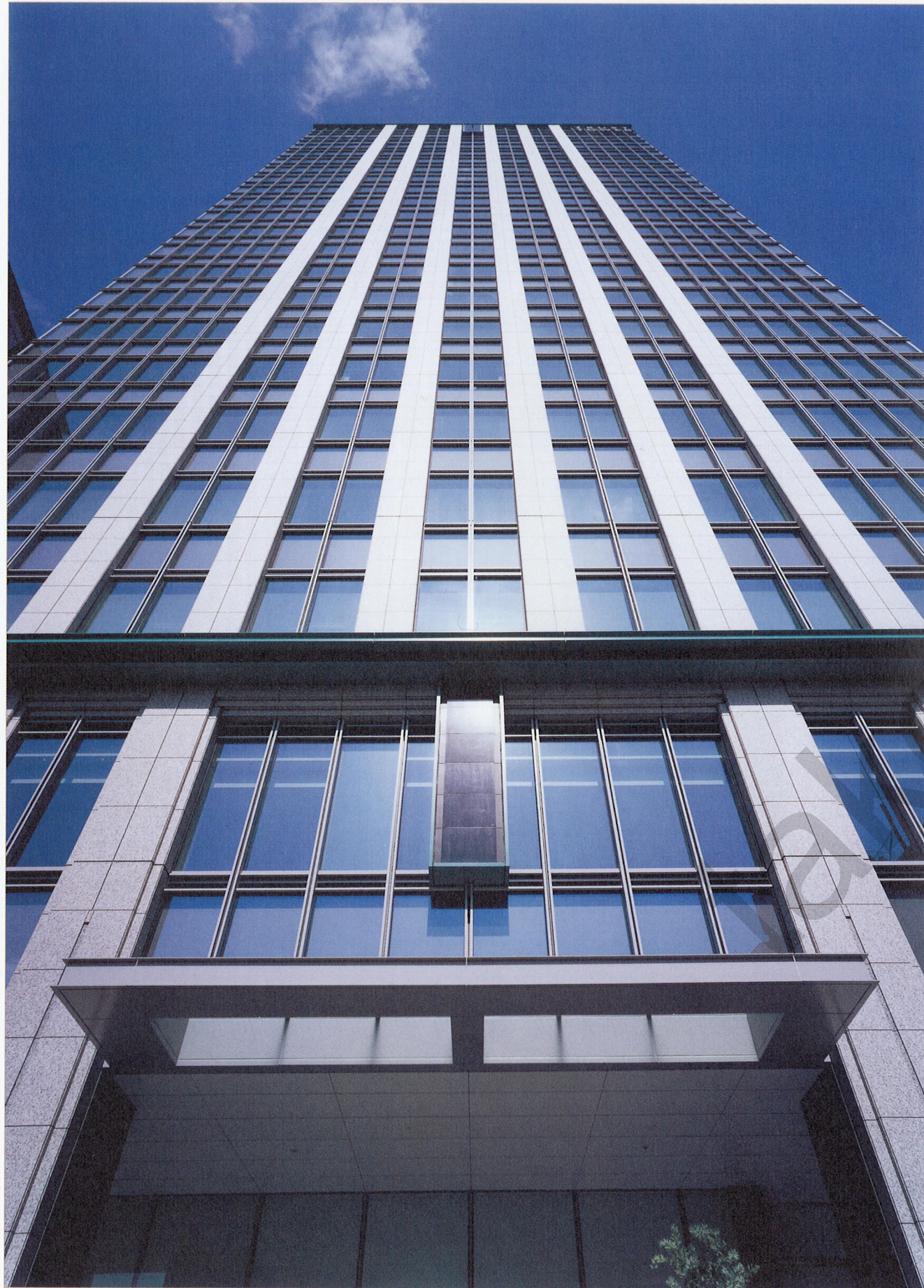
南面より見上げる。6本の白御影石の柱は成長性をイメージ。堂々たる風格の外観。 A view of the new building looking up from the south side. The image formed by the six columns of white granite symbolizes growth potential. A regal presence in a distinctive style.
