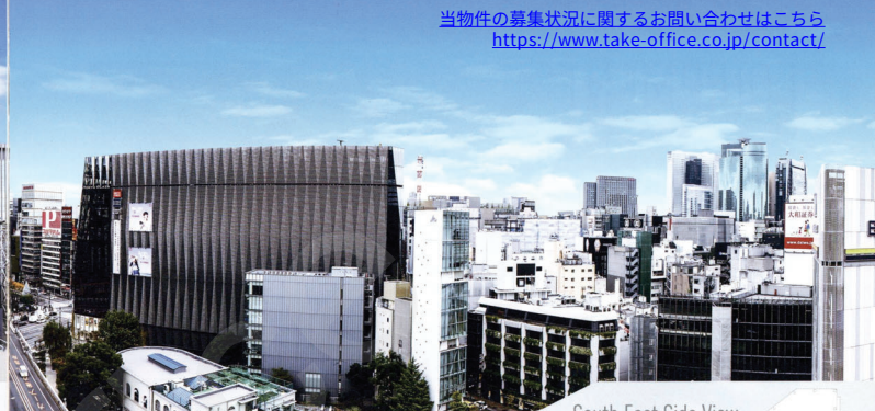
South East Side View
